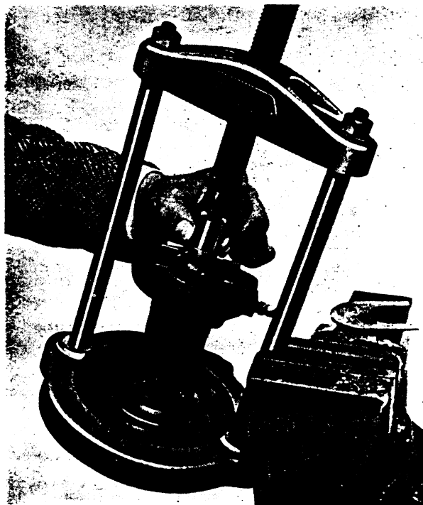
FIG. 12. REPLACING IMPELLOR.
